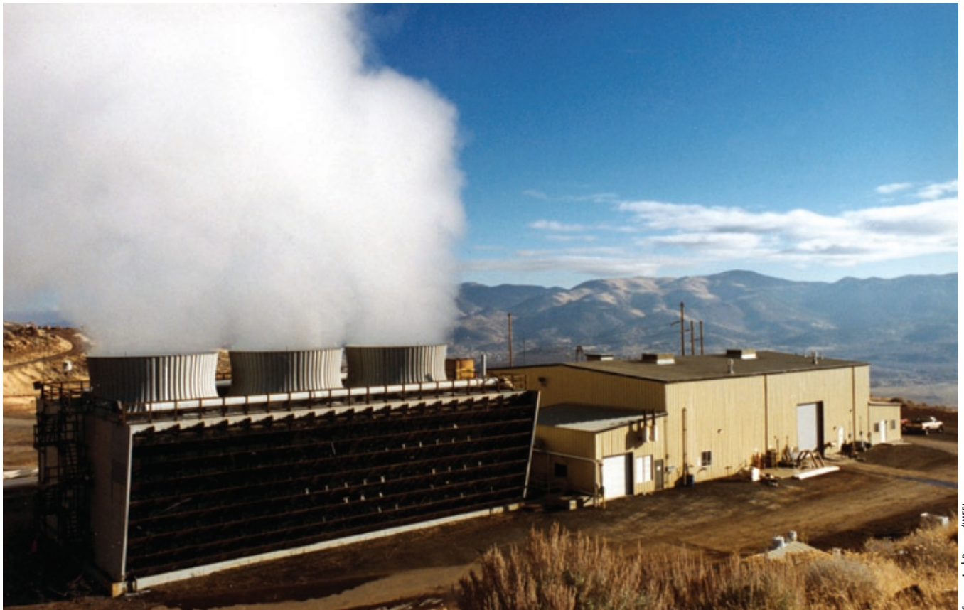
Steamboat Hills geothermal plant, Nevada
