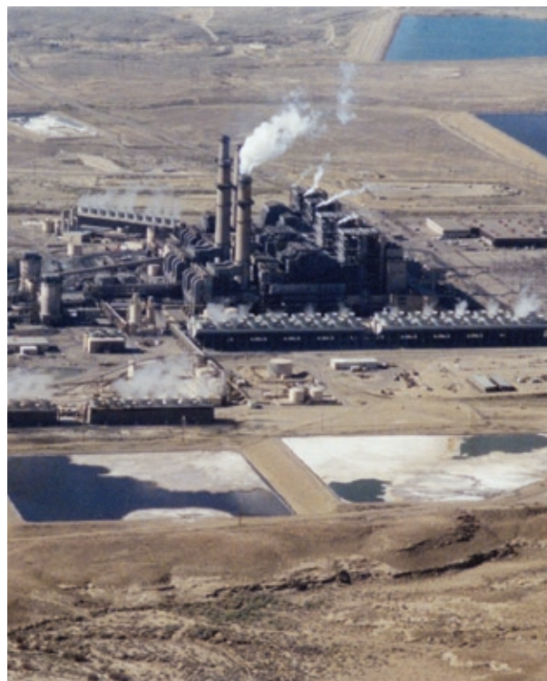
San Juan coal-fired generating plant, New Mexico
