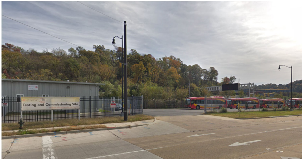
Figure A.7 DC Streetcar Testing and Commissioning Site
