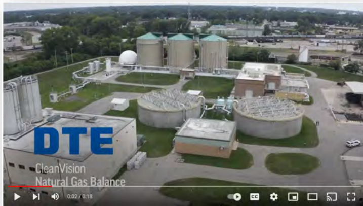
Grand Rapids Water Resource Recovery Facility - Renewable Natural Gas Supply Source
