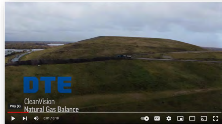
Sauk Trail Hills Landfill in Canton – Renewable Natural Gas Supply Source
